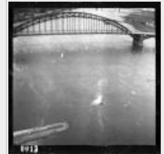
**Through** type - the superstructure of the bridge is entirely above the deck.
