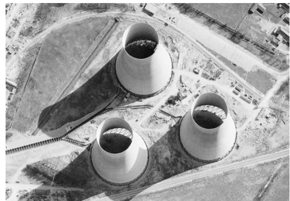
Didcot Power Station under construction, in 1969 (NCAP-000-000-320-583)
