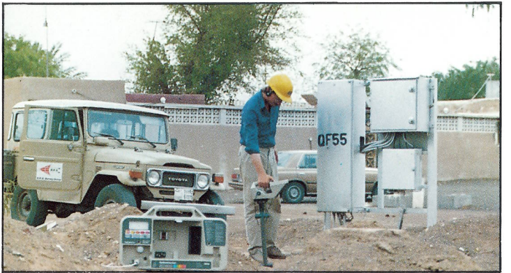
LOCATING UNDERGROUND UTILITIES
