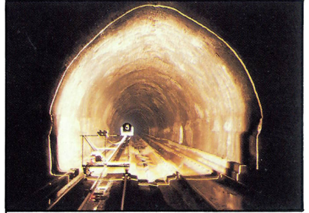
UNITED KINGDOM TUNNEL SURVEYS
