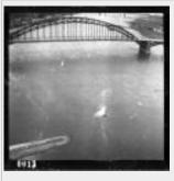
**Through** type - the superstructure of the bridge is entirely above the deck.
